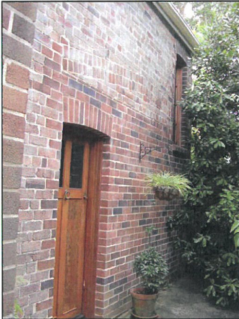
Figure 3.8 The southern façade has undergone some change, infill of early openings and adaption. New windows and door have been added.
